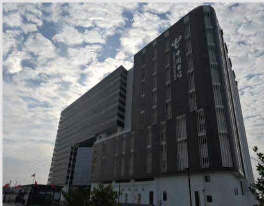
Guangzhou Dongchong Data Center
