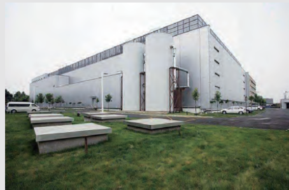
KDDI-Telehouse BeiJing IDC
