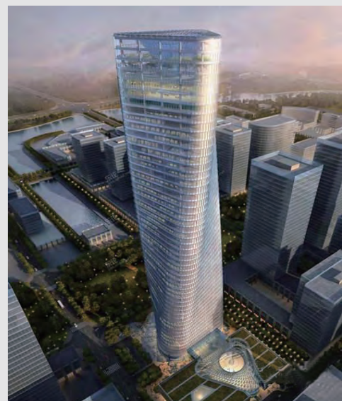
Ningbo Bank of China Building Data Center
