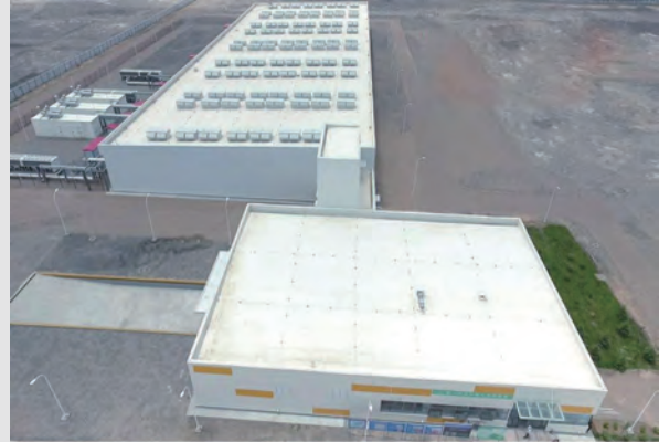
Amazon - Ningxia Zhongwei Data Center
