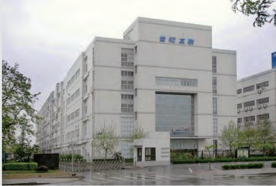
21 Vianet Group Data Center
